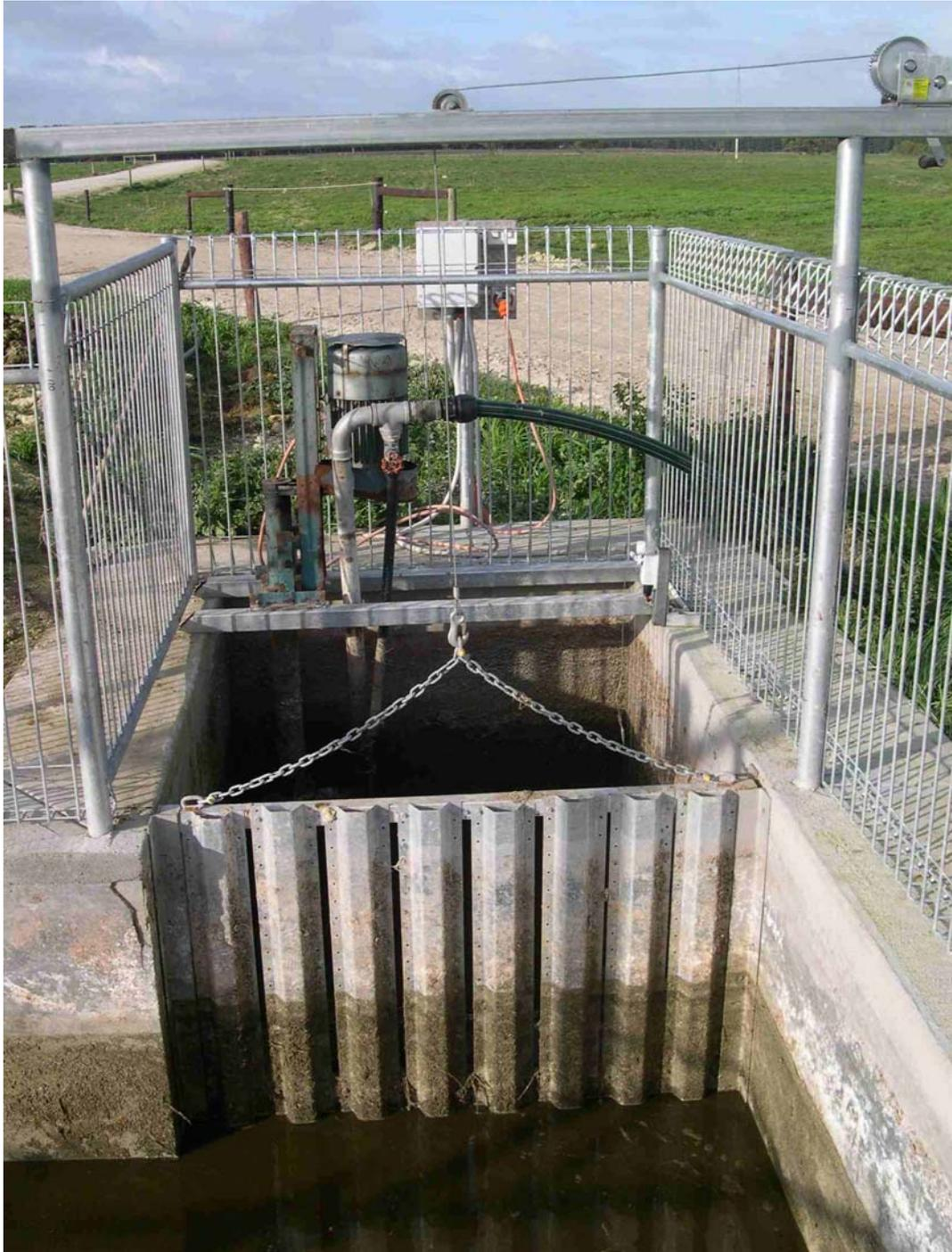
Figure 1. Vertical weir in trafficable solids traps (courtesy of Rural Solutions SA).
