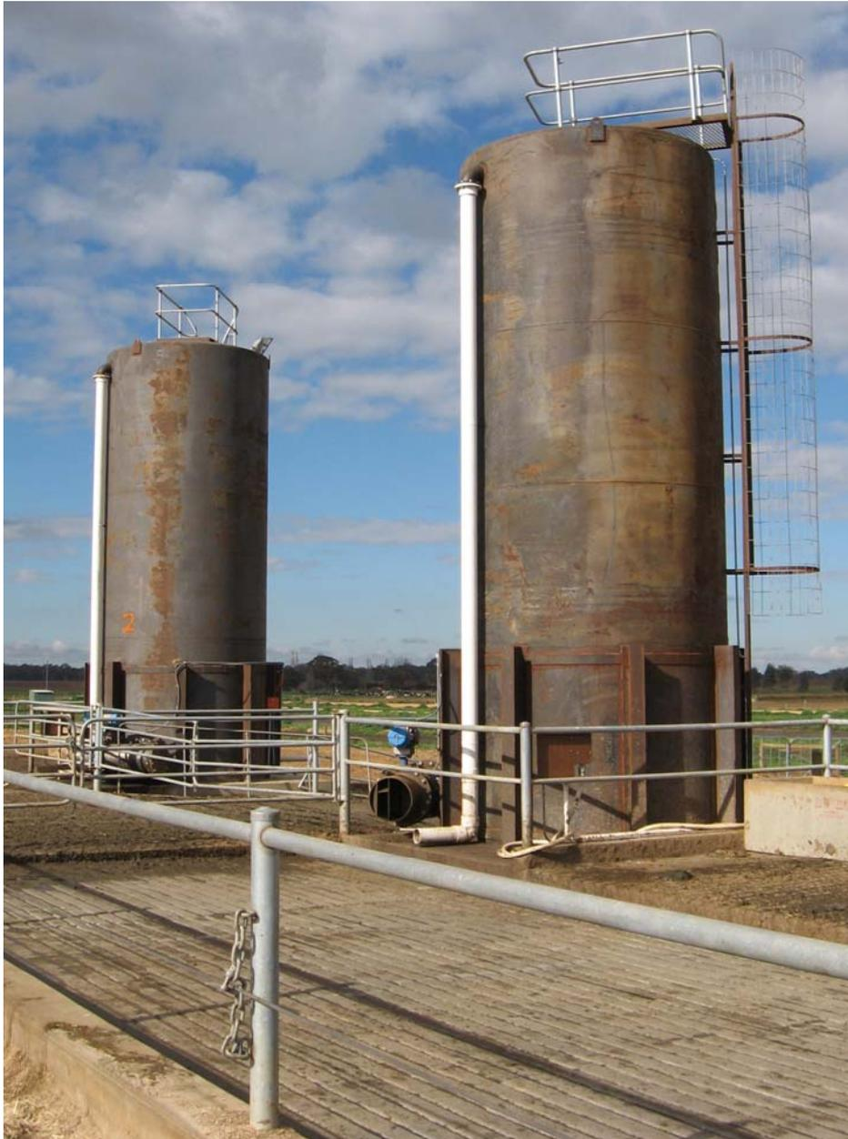
**Figure 1. Floodwash tanks and above-the-surface delivery for feedpad flushing.**
